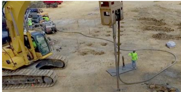
Pile installation and material handling equipment
