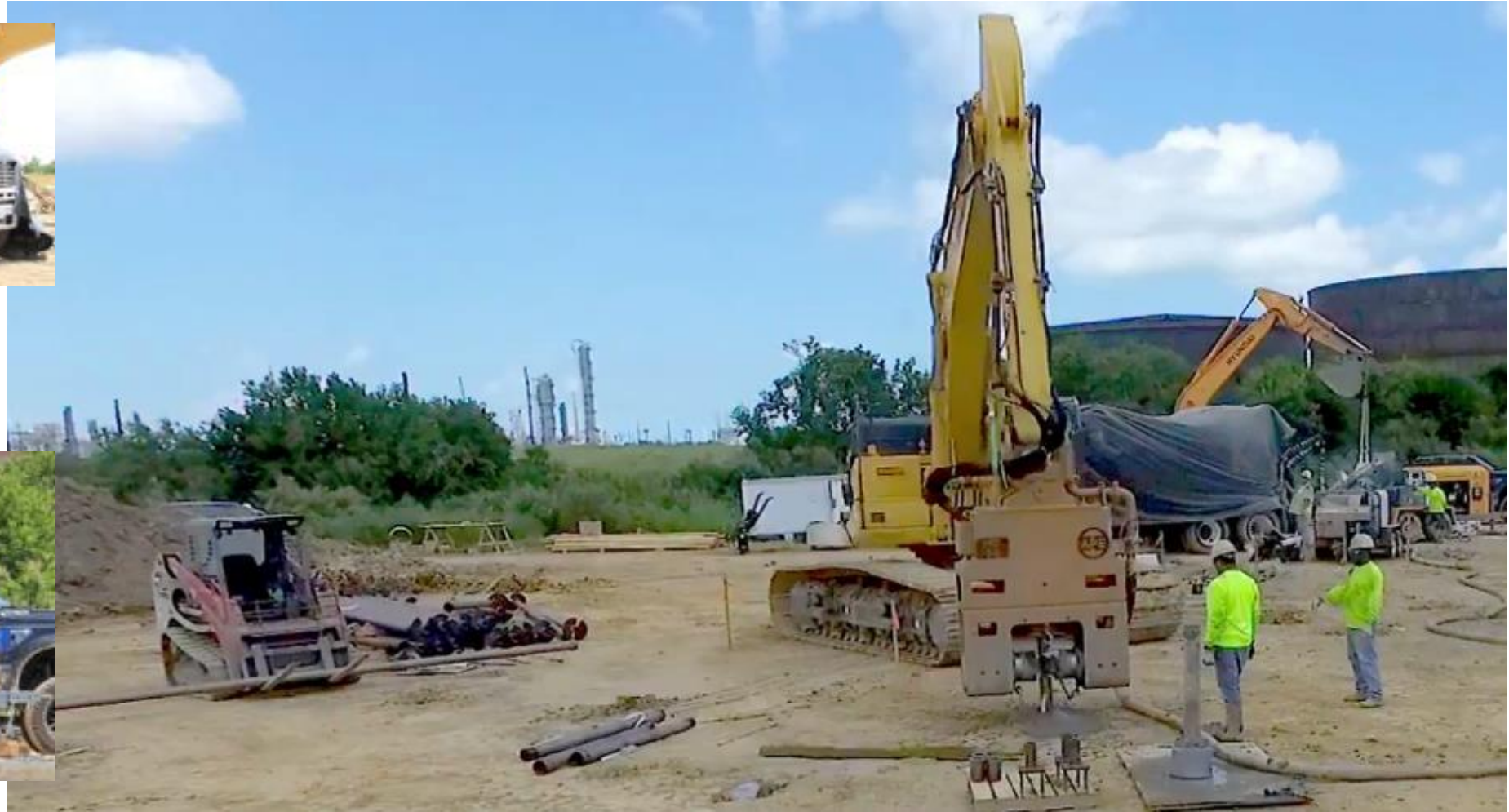
PILING INSTALL AND MATERIAL HANDLING EQUIPMENT
