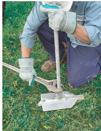
1. Thread a standard anchor rod into the threaded shackle of the Manta Ray® anchor.
