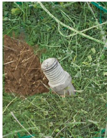
4. The end of the anchor rod should be at ground level. (In looser soils, may be countersunk up to 12" below the surface for greater holding capacity.)
