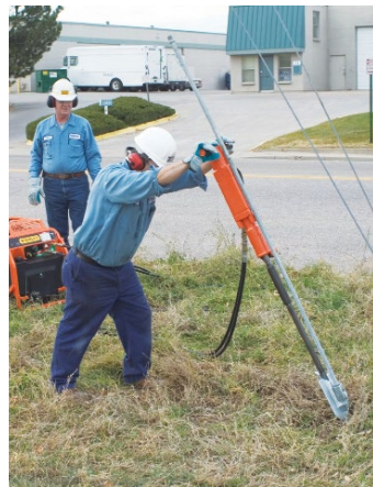
2. Insert drive steel into the anchor. Position and angle.
