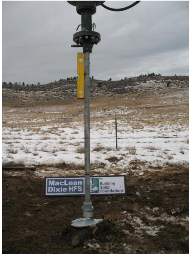
Installing RCS (Round Corner Square) Tension Anchor
